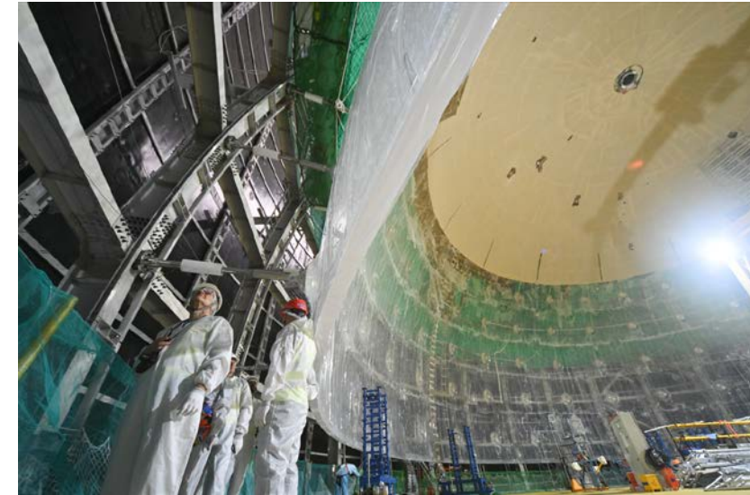
Acrylic sphere from top to equator layer (1/2 completed)
