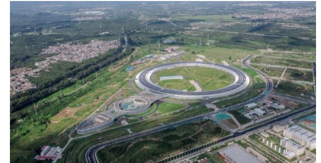
HEPS photovoltaic power capacity of 10MW
