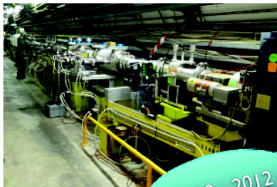
UA9 installation in the SPS
