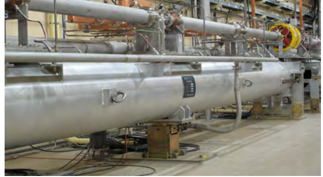
Figure 9: New support table installed for restricting the displacements of the girder unit in both the transverse and axial directions.
