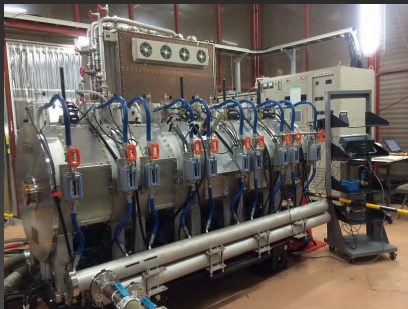
5-gap FT3L cavity in Hendel test bench.
