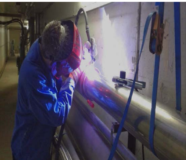
Cold piping constructed and installed by Demaco
