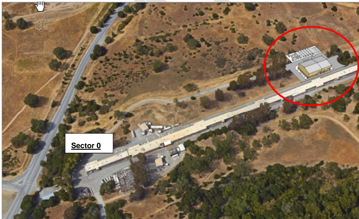
Figure 11-2. Cryoplant location at Sector 4
