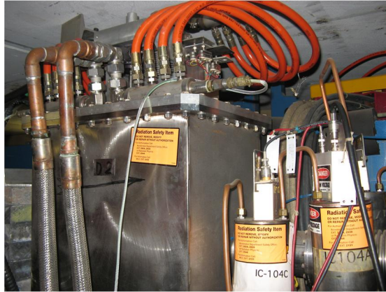
Figure 5-68: Existing D2 in BSY tunnel
