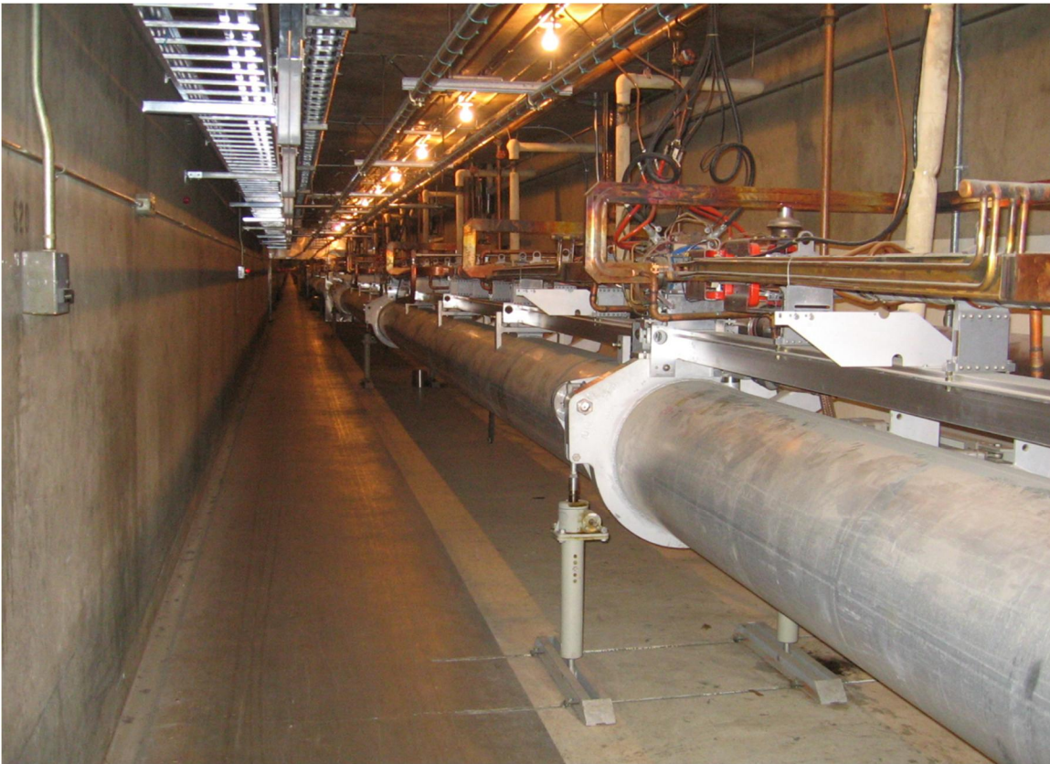
Figure 11-3. Accelerator Equipment to be removed from SLAC linac Sectors 0-10, 1,000 meters
