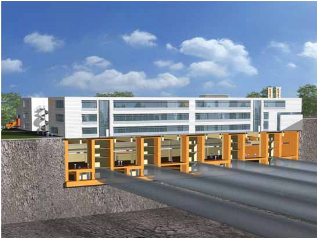
Figure 7.1.28 Three-dimensional view of the experimental hall and laboratory complex as viewed from the incoming photon tunnels XTD6-10.
