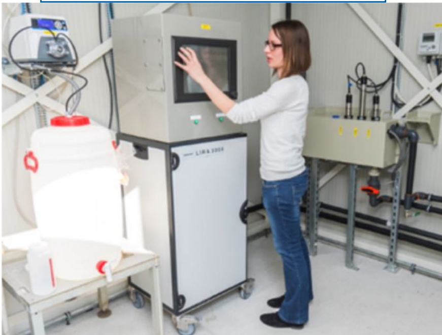
Water monitoring station WMS – CERN SMART
