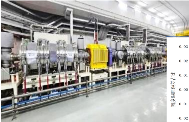
Cavities in tunnel
