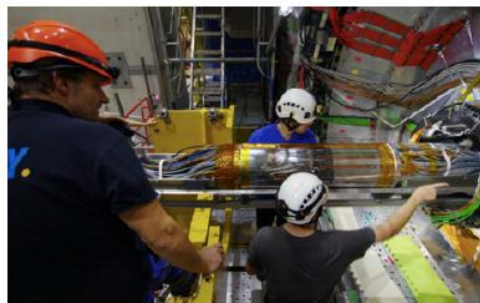
Installation of VXD
