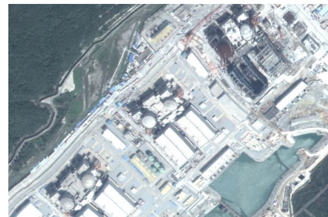
Yangjiang Power Plant
