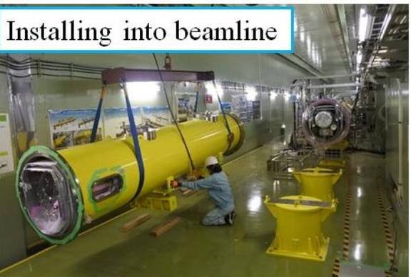
Installing into beamline
