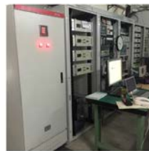
Modulator and klystron
