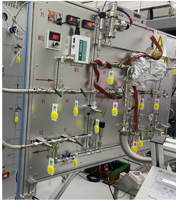
Gaseous source injection panel
