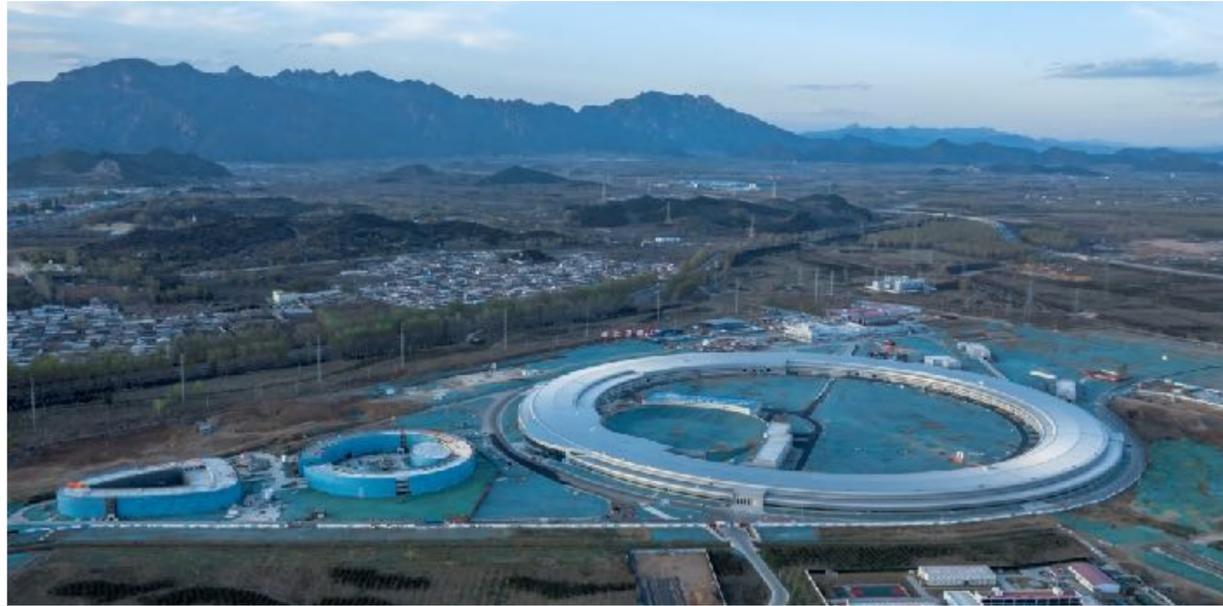
beam energy 6 GeV, 1.36KM,  $\leq 0.06\text{nm}\cdot\text{rad}$ , 14 beam lines
