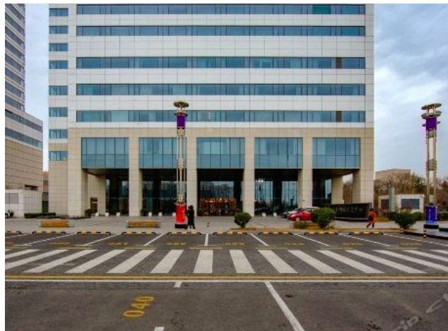
Figure 6: Hi Chance (Dalian) Science & Technology Center
