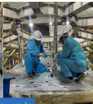
Connecting bar to acrylic node
