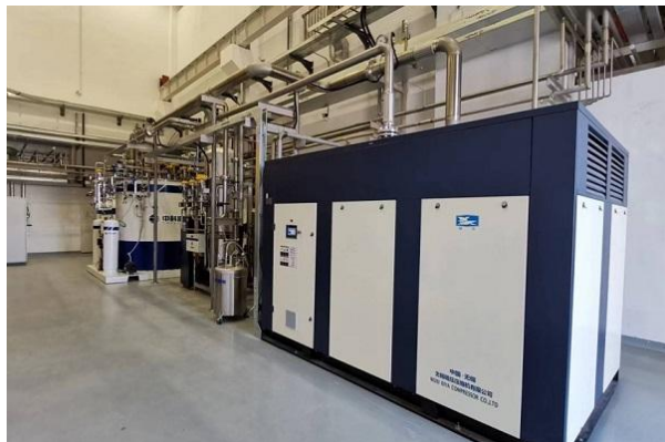
China company made 850kW@4K cryogenic plant installed in IHEP South Light Source test facility in Dongguan (May, 2022) (Next step is 10~18kw@4K)
