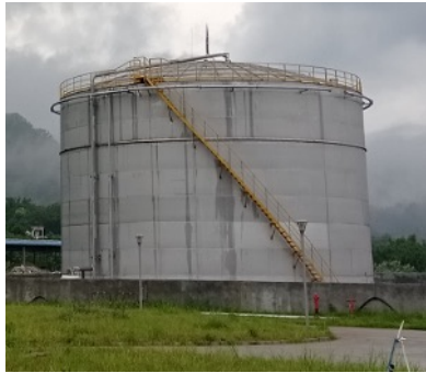
5000 m 3 LAB tank
