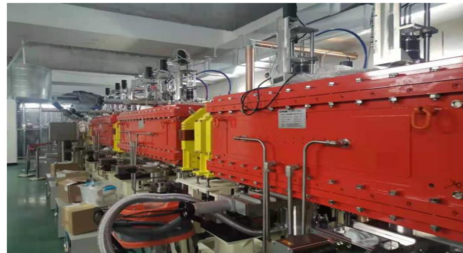
Cavities in tunnel
