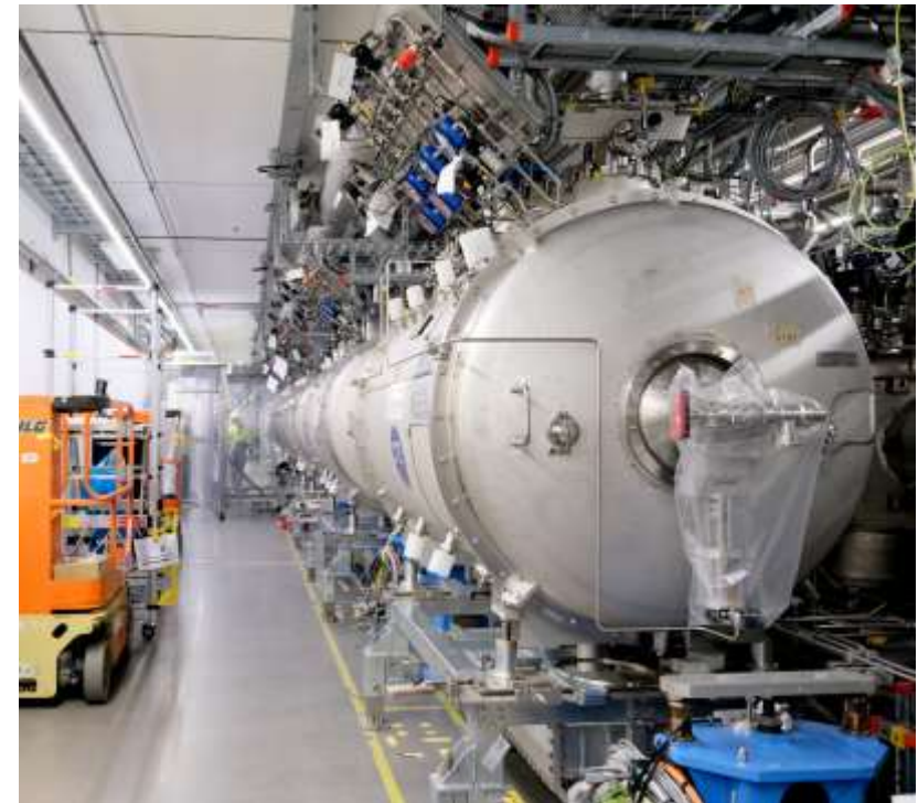
Spoke Cavities being installed
