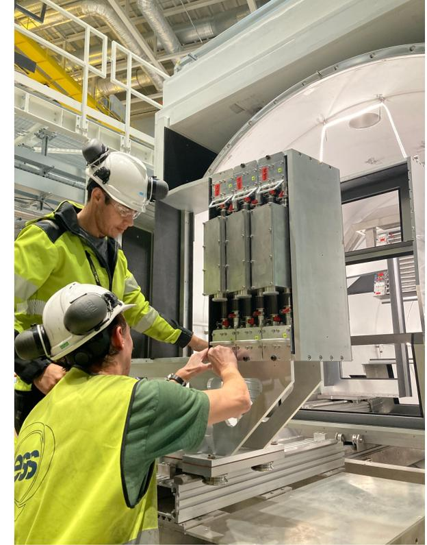
**Installation of the front and middle panel detectors at ESS**
