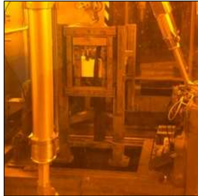
Images of the remote handling work in the cell to strip out old TRaM assembly
