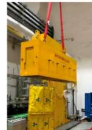
Used shutter insert removal & storage Net time for replacing a set of Shutter Insert is ~4.5h
