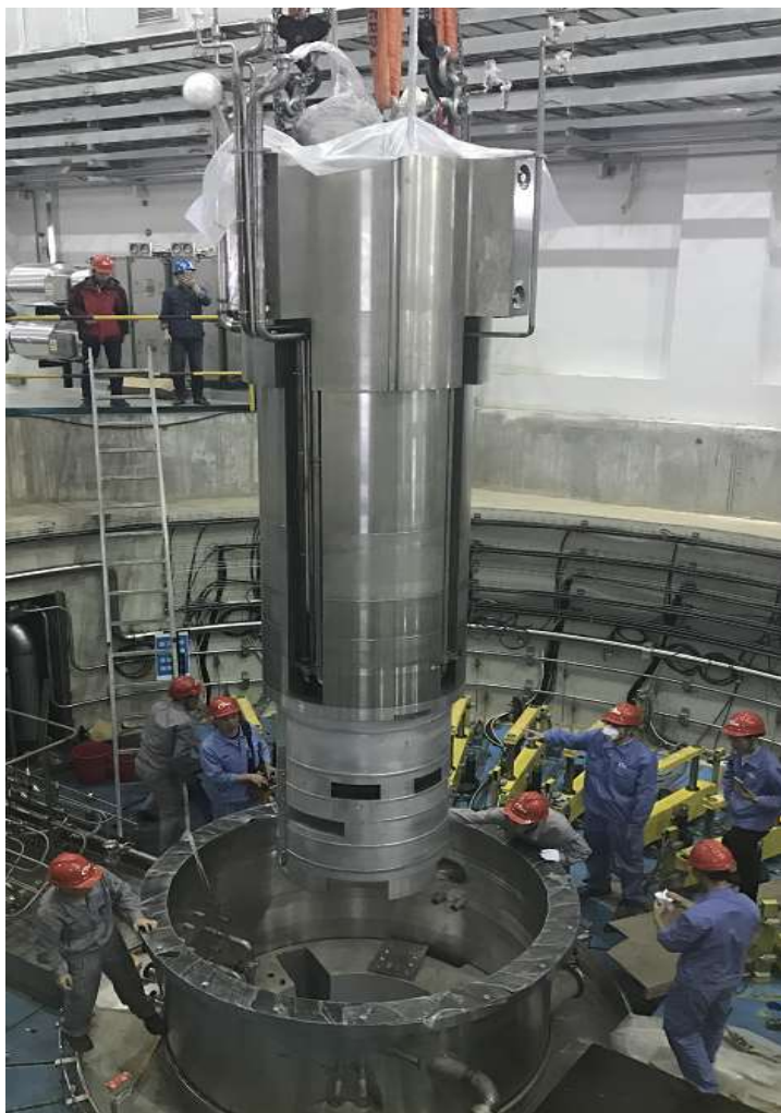
MR plug@~33tons and 5.4m height
