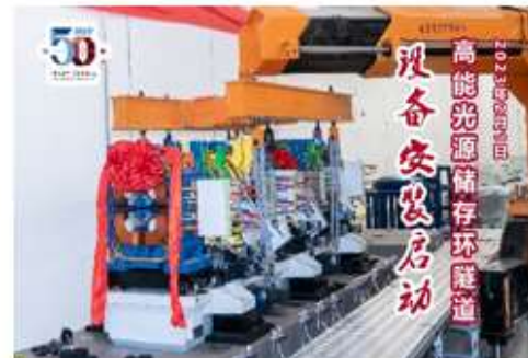
Feb. 1, 2023 The first girder was installed in the storage ring tunnel
