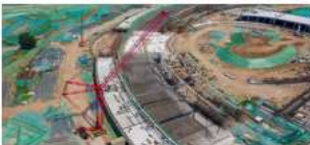
July 1, 2020 The first steel beam was installed
