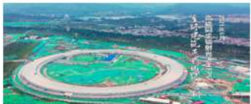
June 27, 2021 Roof-sealing work for the main ring building completed
