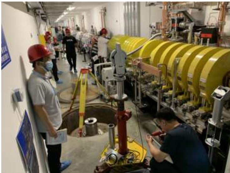
Smooth precise alignment of linear accelerator
