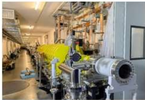
May 12, 2022 The Linac Vacuum-sealing in the tunnel completed
