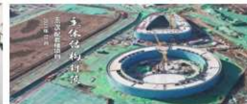
Nov. 18, 2021 Roof-sealing work for ancillary buildings completed
