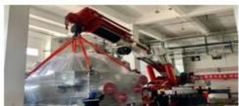
Apr. 13, 2021 Utility installation in NO.2 Hall commenced
