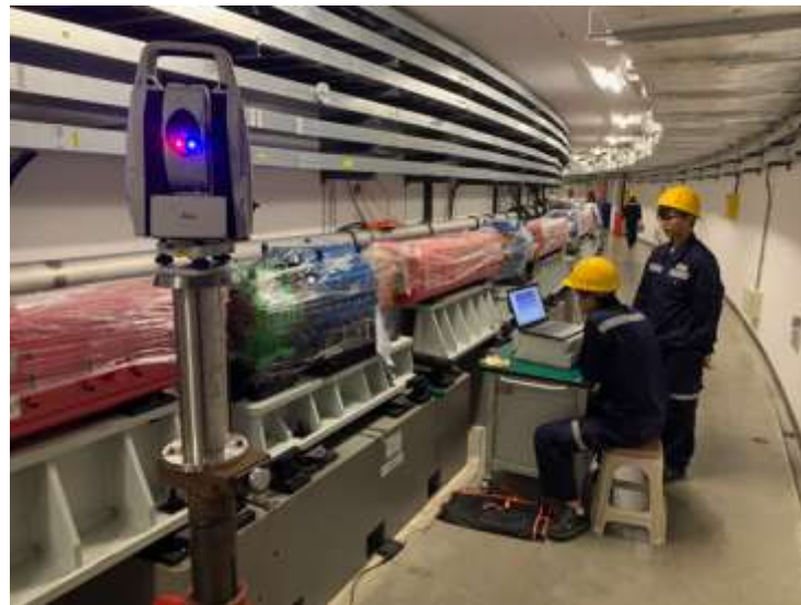
Smooth precise alignment of booster
