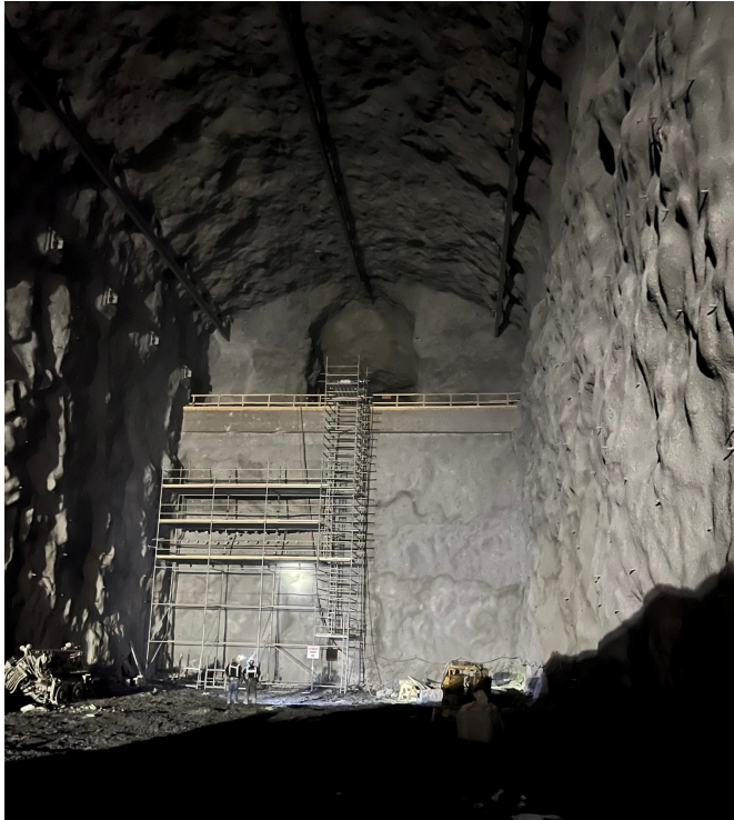
East end scaffolding progress in South Cavern
