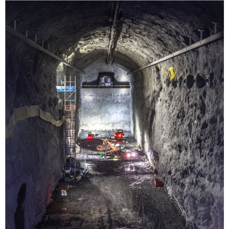
Concrete work underway in North Cavern
