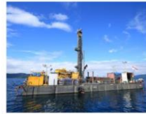
Drilling work on the lake
