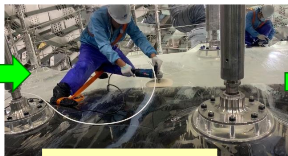
Bonding line sanding
