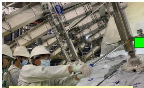
Supporting bar installation
