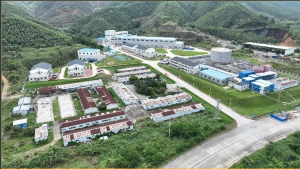
Juno Experiment Campus, Kaiping, Guangdong
