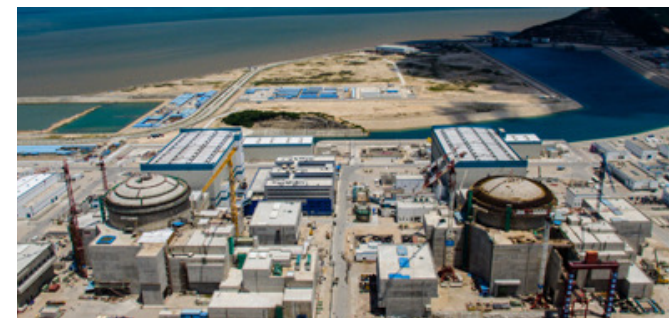
Taishan Power Plant
