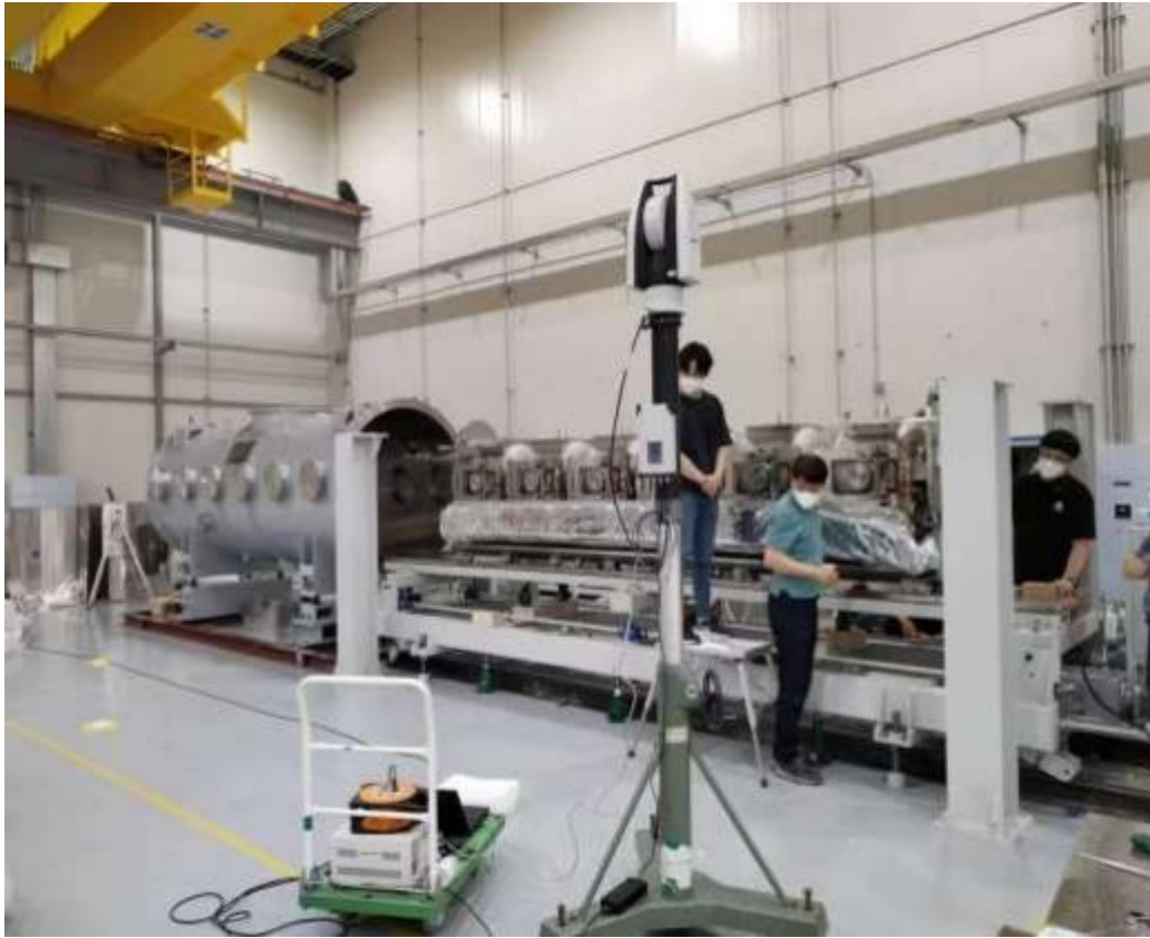
Cavity string alignment
