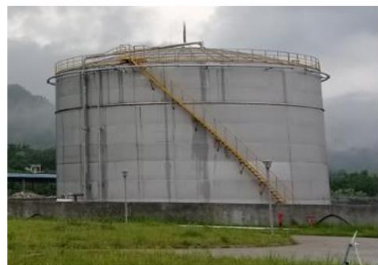
5000 m 3 LAB storage tank
