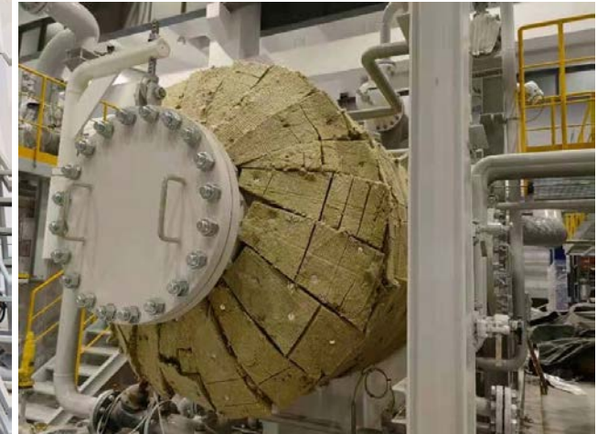
Insulation installation
