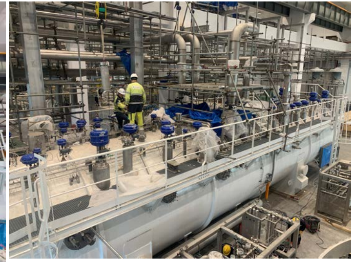
Main components installation
