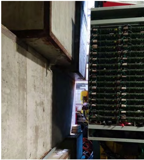
1 HV mainframe HV patch panels
