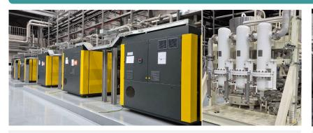
Compressor (HP+LP) & Oil Removal System (Warm Compressor Section)
