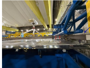
first installed TT wall
