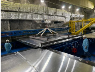
first installed TT wall
