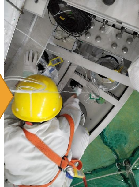
Install Light Barrier
