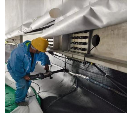
Welding on the wall
