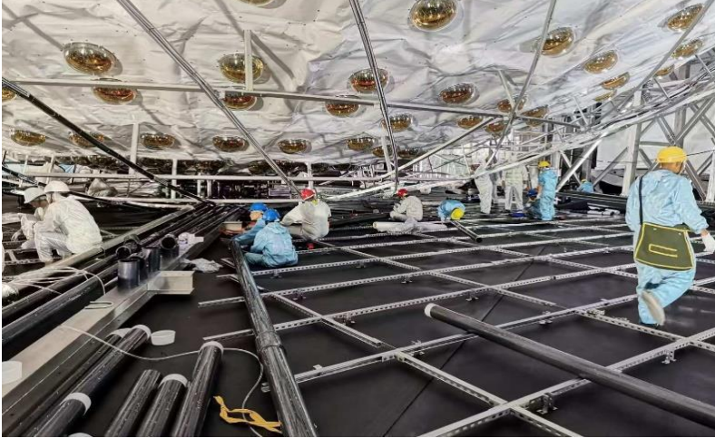
Assembling the Unistrut support structure
