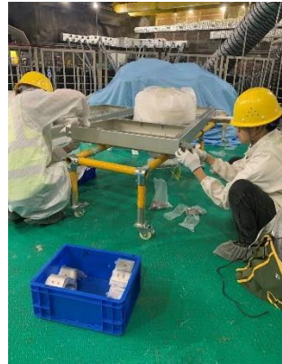
Install PMT/electronics box
