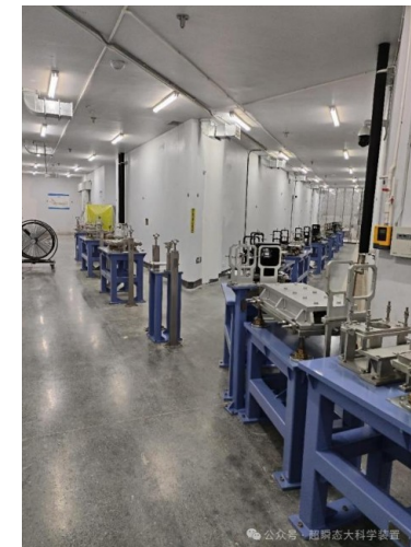
Beam transport line
