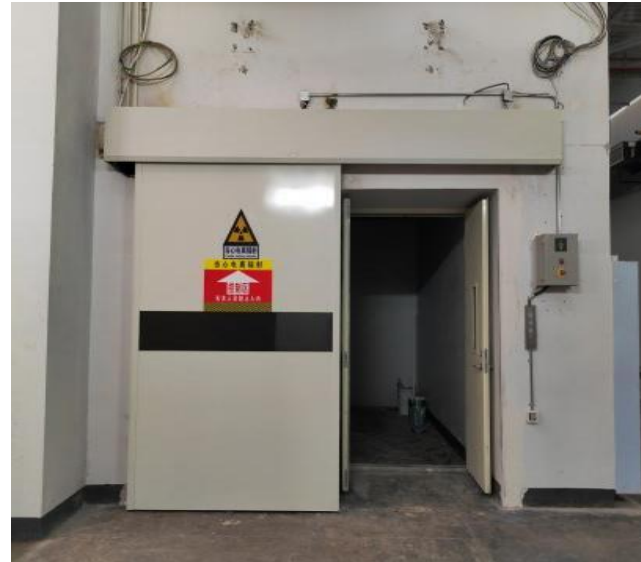
Shielding door in linac
