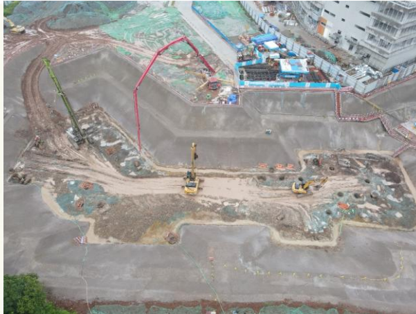
Excavation & Foundation Work of Linac
