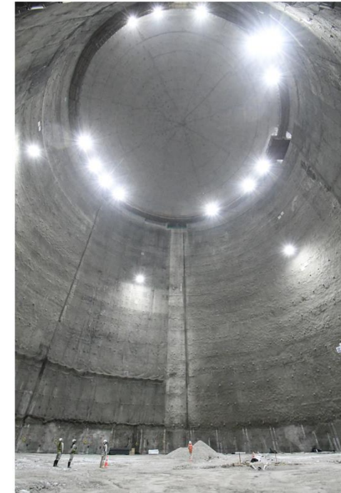
Hyper-Kamiokande, 600 m underground.
