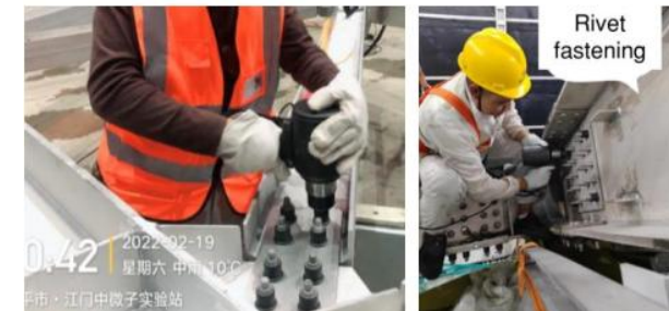
Bolts and riveting
