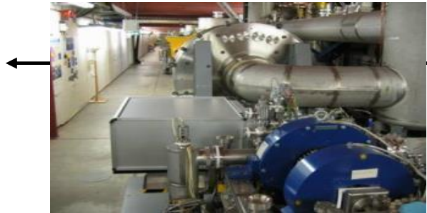
Normal conducting 1.3 GHz RF gun Cs 2 Te cathode / 5 injector lasers
