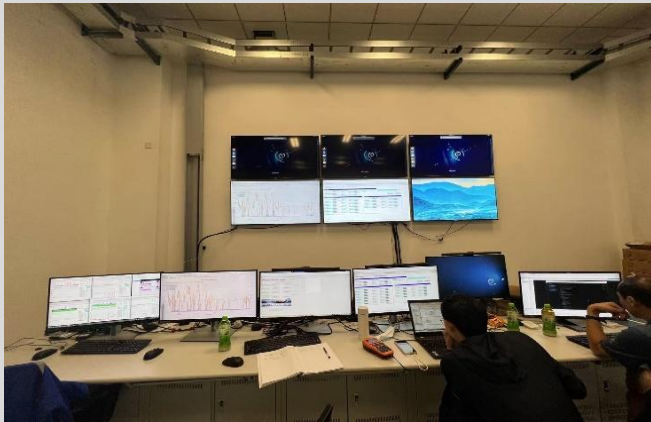
Temporary Linac Control Room
