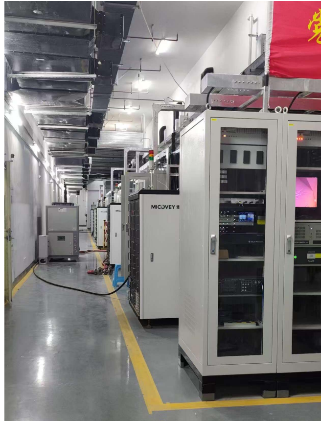
Service tunnel (Feb. 2026)
