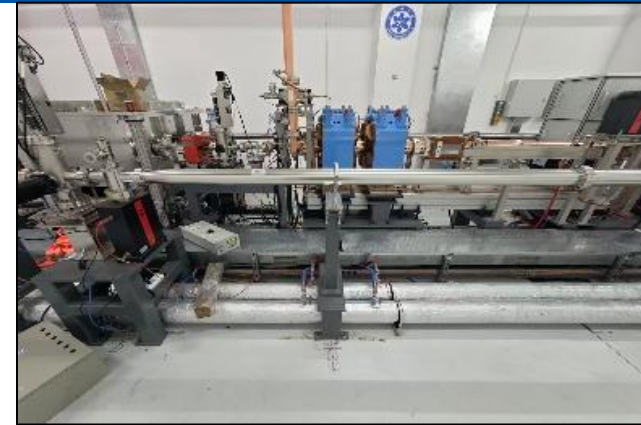
Site before chamber installation
