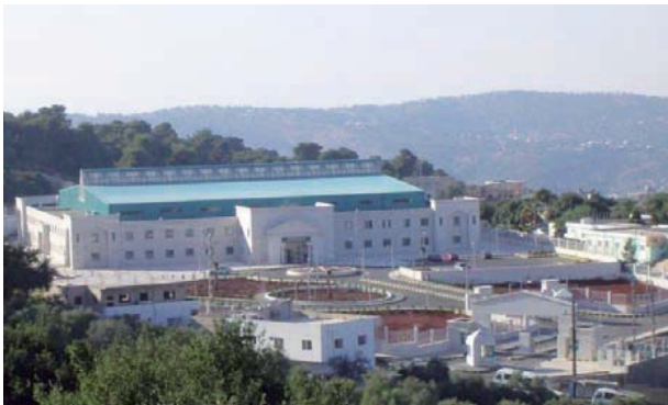
Figure 1: The SESAME building
