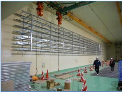
**Figure 1.** Part of the existing fiducials were hidden by conventional equipment (cable trays).
