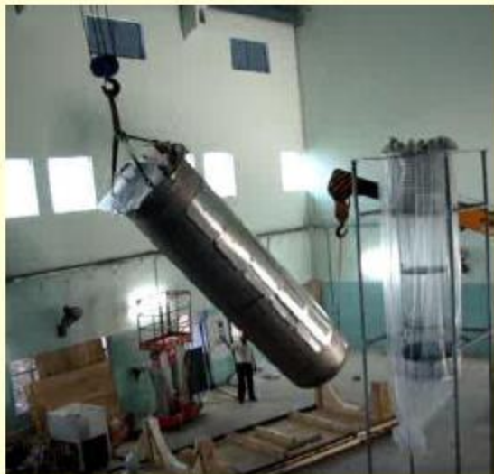
Installation of cryostat in pit
